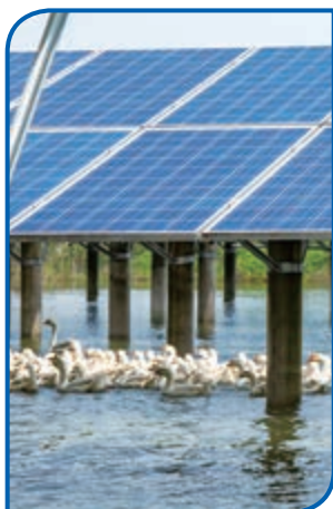
Fanchang Fishery-PV Power Plant 繁昌漁光互補電站
